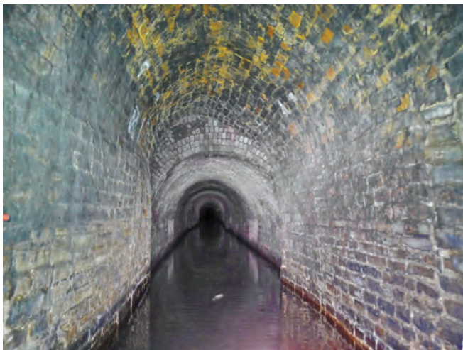
Original brick lining from the 1795 tunnel work.
